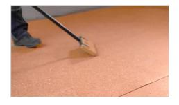
By rolling over the entire surface with a 50kg roller when installation is complete
